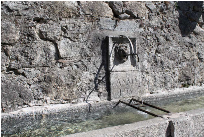
Fig. 5 Waterbak in Santa Croce
